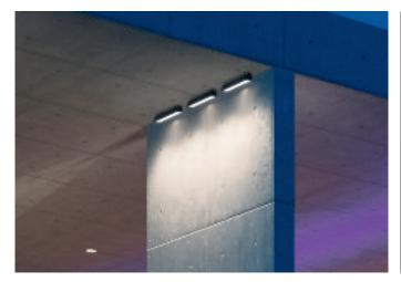
When mounted in a row along the building, the broad light distribution and its even gradient ensure uniform facade illumination
