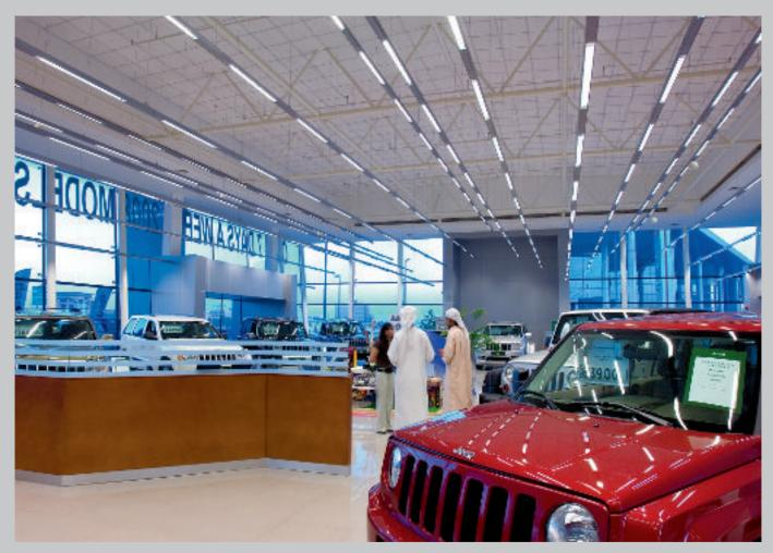
The T16 light structure is identified by its very precise design. Due to its compact dimensions it is an inconspicuous architectural detail. It's versatility as a lighting tool means it can be used universally. T16 light structures are designed primarily for the T16 fluorescent lamp. They are always suspended at the ends of the profile so that unsupported spans of up to 3.2m are possible.
