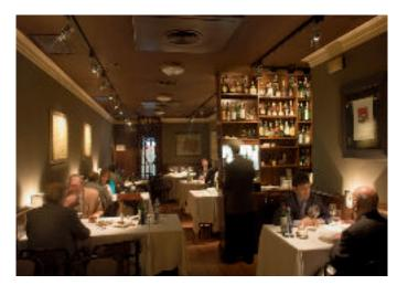
The system philosophy behind these luminaires provides solutions for different lighting concepts in one luminaire range: narrow to medium light beams for accent lighting and lens wallwashers for the uniform illumination of shelves or walls. The projection spotlights with framing attachments are suitable for the illumination of pictures to give the impression of the pictures being illuminated from within.
