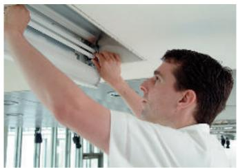
The coloured light from the TFL wallwasher is produced by three coloured 28W T16 fluorescent lamps. A light colour mixer consisting of a combined reflector-diffuser system ensures an even, totally mixed light which is projected onto the cover glass without any coloured shadows. Due to the spectral properties of coloured fluorescent lamps, all the colours of light produced have a pastel character.
