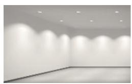
Downlights with narrow diffusers are used for example, for ambient lighting in rooms with ceiling heights of more than 3m.
